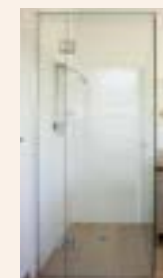
SHOWER SCREEN LOCATION: ENSUITS & BATHROOMS DESCRIPTION: FRAMELESS GLASS SHOWER SCREENS. FROSTED GLASS IN MASTER EN-SUIT.
